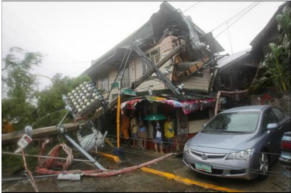
A house along Antipolo street in Tondo, Manila is badly damaged by an electricity post that was felled by strong winds brought by Typhoon Pedring. Photo by Rem Zamora for abs-cbnNEWS.com
